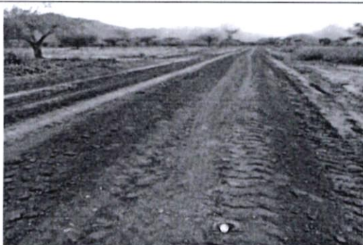
Figure 1: Kacheliba-Nakwapuo-Cherangan road grading
