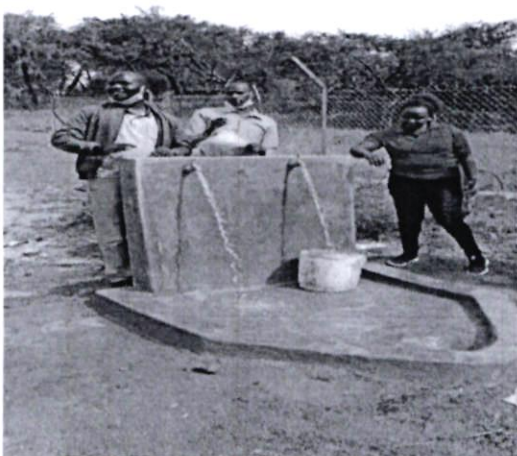
Figure 5: Newly Upgraded Lokitonyala Borehole
