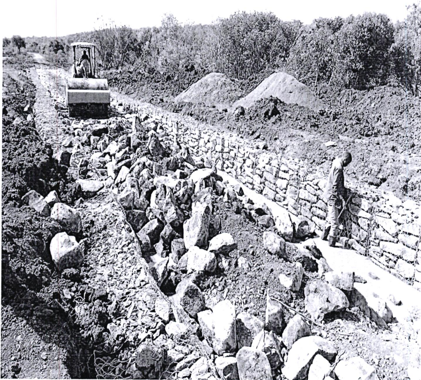
Improvement of Poro-Loosuk-Suguta Marmar Road
