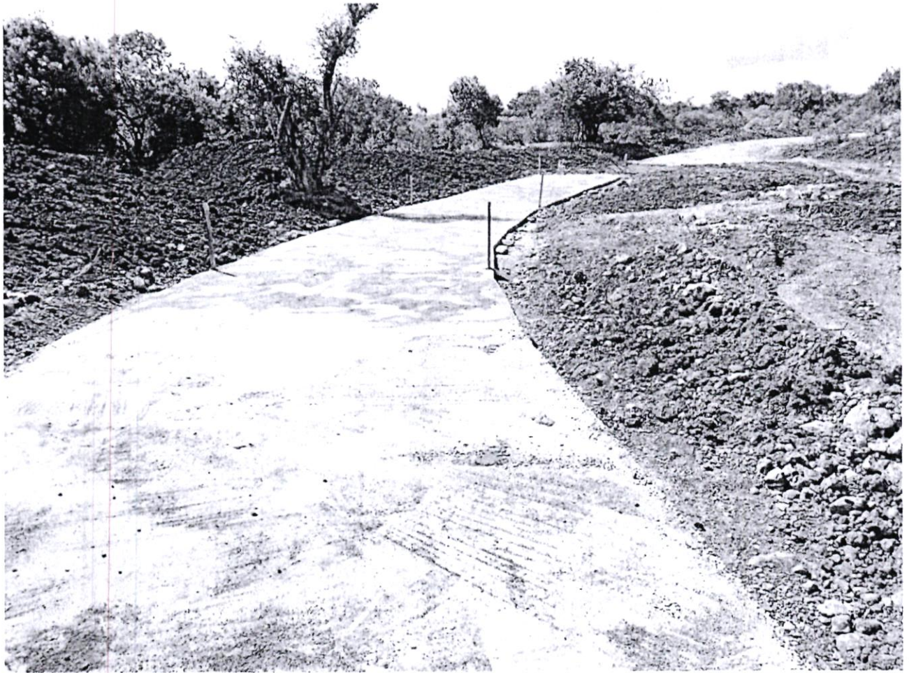
Installation of cross culverts and construction of level drifts
