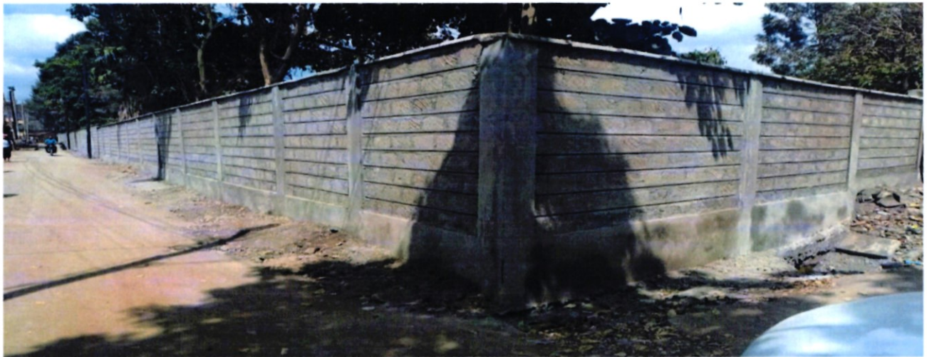
Project 1: Construction of Perimeter Wall at Kawangware Primary School
