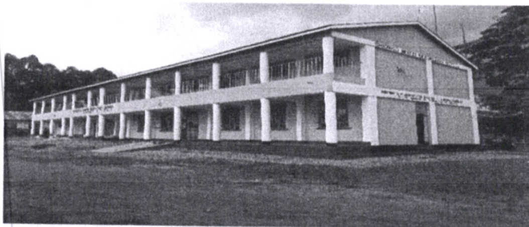
Shiongo Mixed Secondary School - Construction of a storey building comprising of Administration office and 4 no.classrooms.Complete, handed over and in use.
