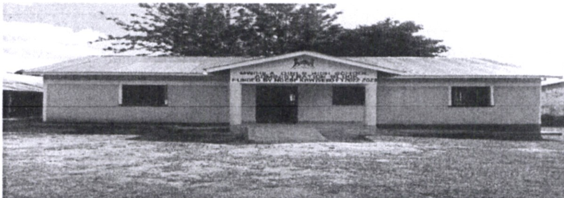
Mwihila Girls Secondary School - Construction of an administration block - Complete, handed over and in use.
