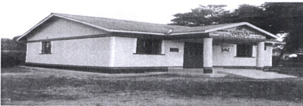
Emutsasa SubLocation - Construction of Assistant Chief's office - Complete, handed over and in use.
