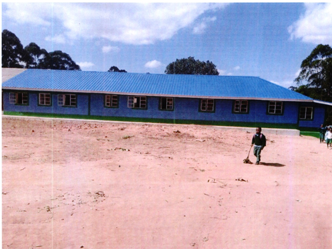
FIG 2: KAVUTINI PRIMARY SCHOOL-RENOVATION
