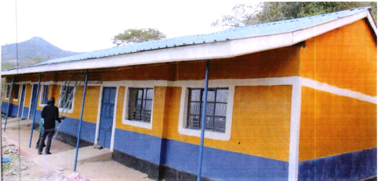
FIG 1: KATULYE PRIMARY SCHOOL-RENOVATION
