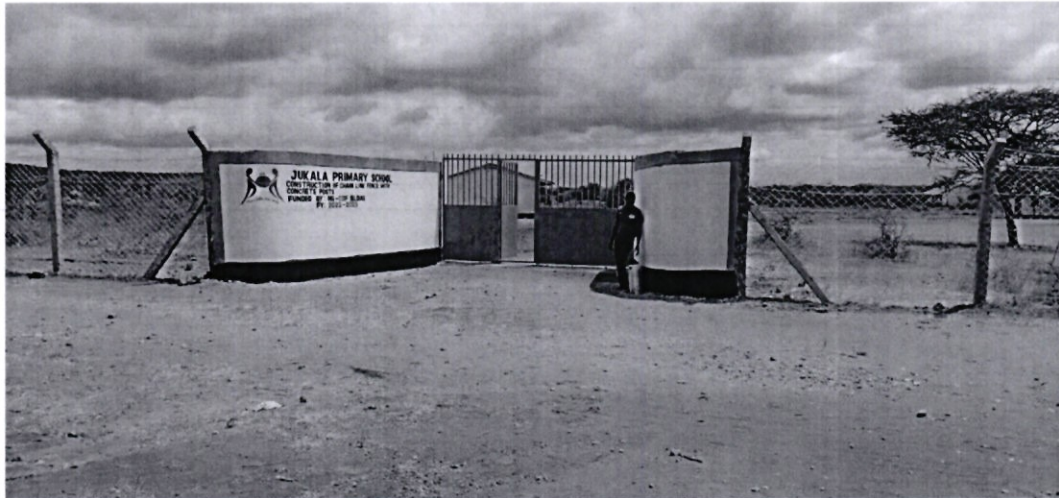
Jukala Primary School-Construction of fence
