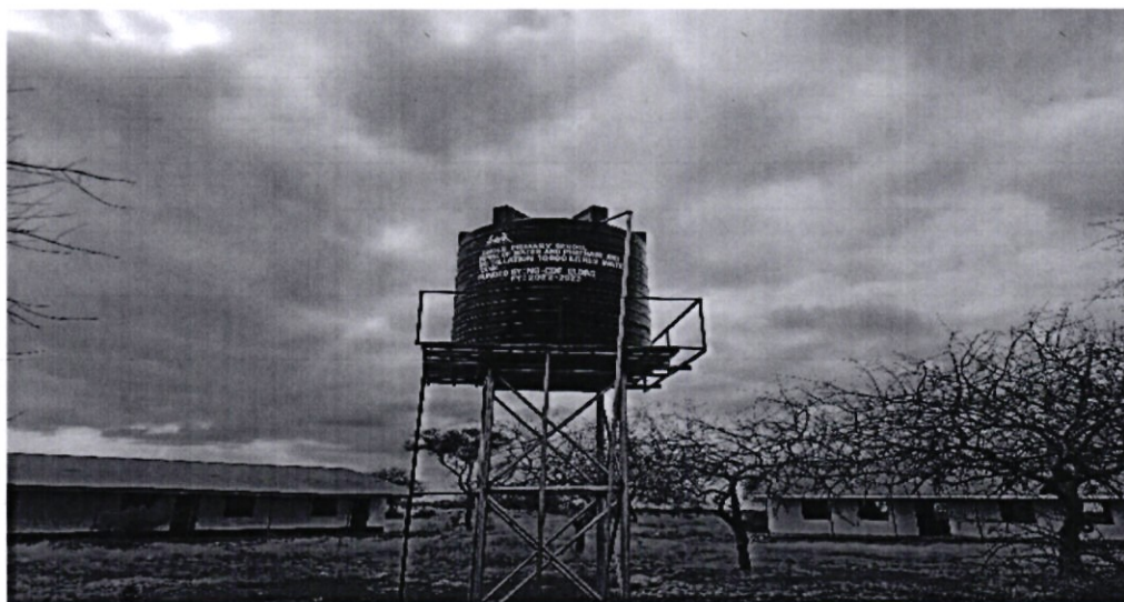
Anole primary School-Piping of water and installation of water tank
