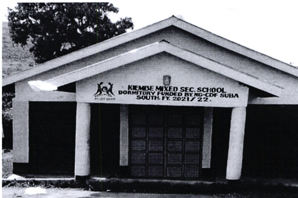
Kiembe Secondary School: Construction of 100 capacity dormitory. Funded: Allocation Kshs 3,400,000 FY 2021/2022
