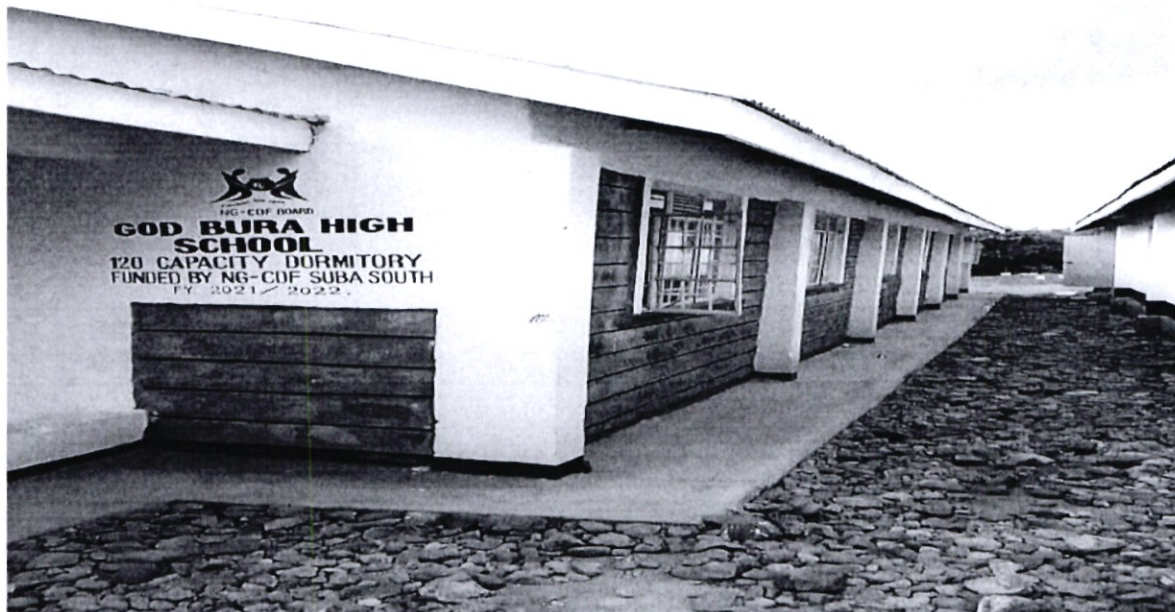
God Bura Secondary School: Construction of 120 capacity dormitory: Allocation Kshs 4,000,000 FY 2021-2022
