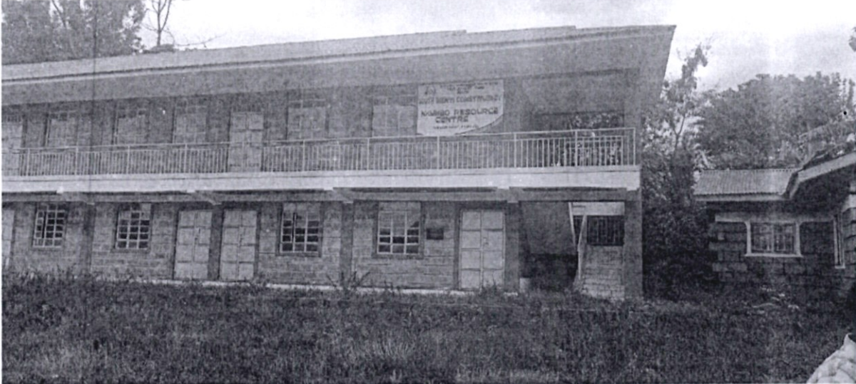
Photo3: Newly Constructed Nkumbo Resource Centre in Nkumbo Location
