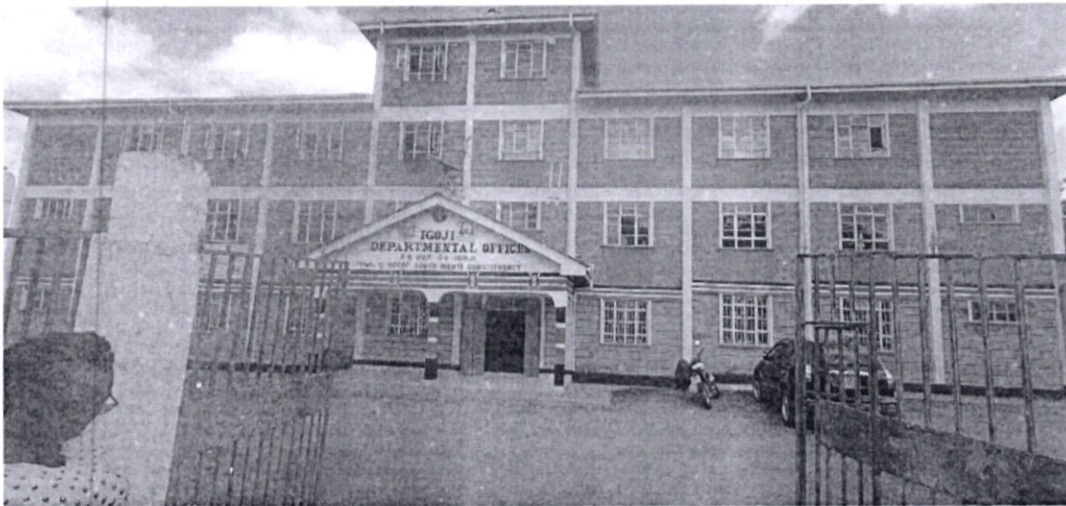
Photo 1: Igoji Departmental Offices Building Comprising of 28 Offices at Igoji Township
