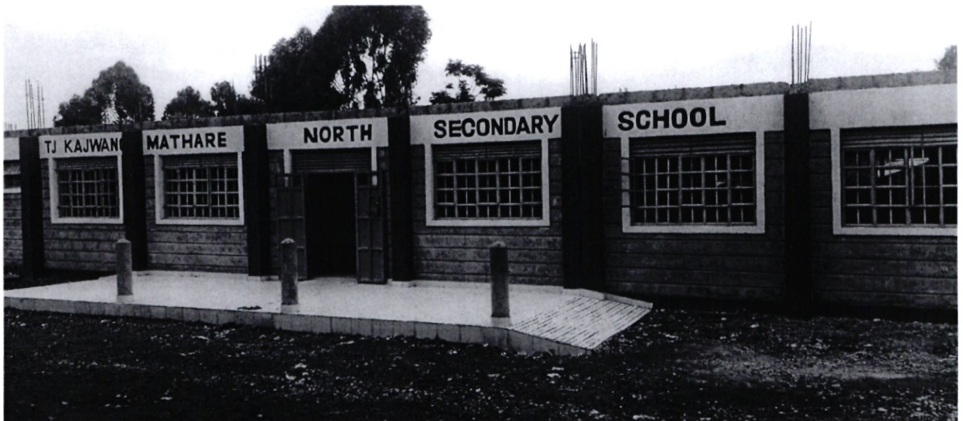
Construction of TJ Kajwang Mathare North Secondary School
