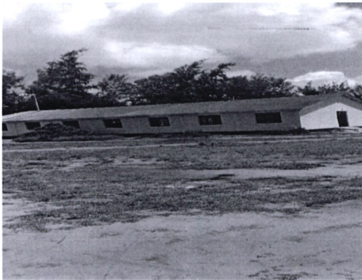
Msambweni Secondary School (Construction of a Multipurpose Hall)
