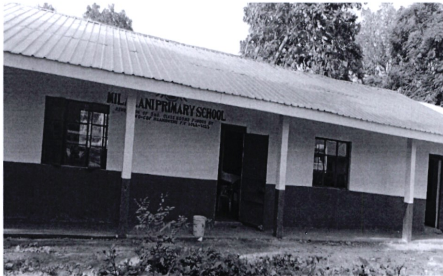
Milalani Primary School (Renovation of 3 Classrooms)
