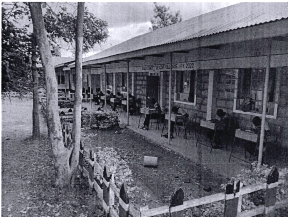
Oldonyo Orok Secondary School; 2 classrooms constructed
