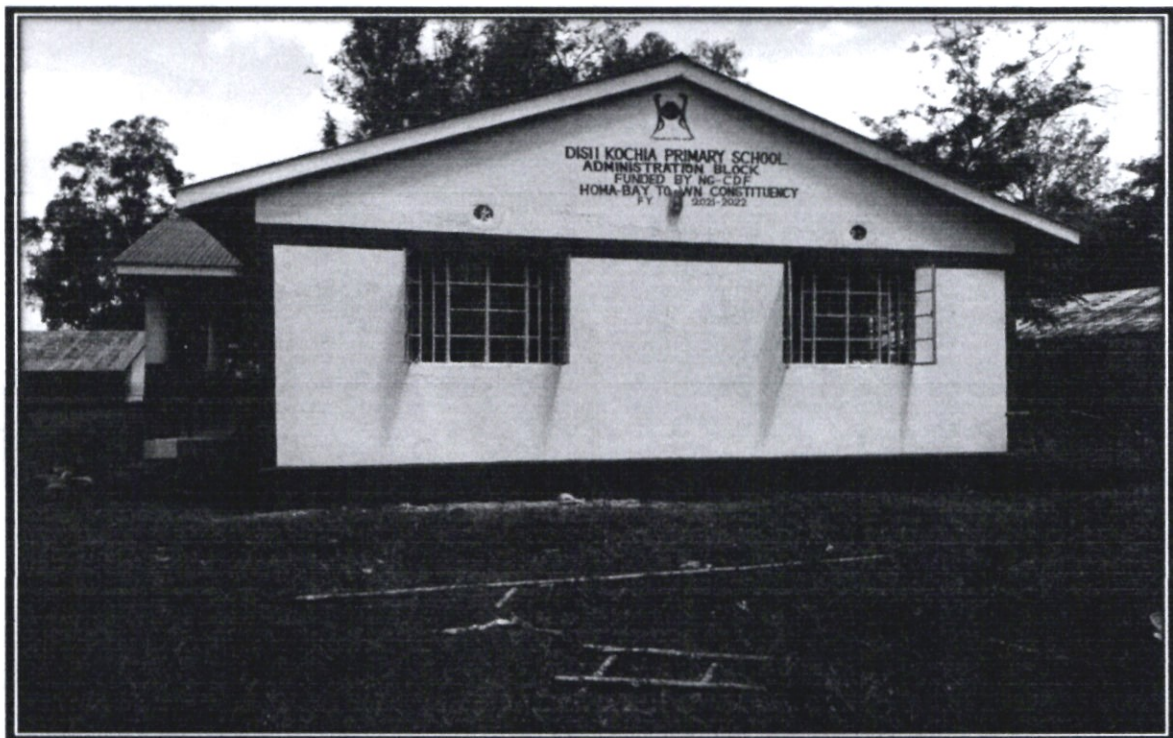
DISII PRIMARY SCHOOL: CONSTRUCTION OF AN ADMINISTRATION BLOCK
