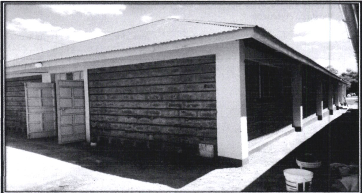
OGANDE GIRLS HIGH SCHOOL: CONSTRUCTION OF A DORMITORY HALL
