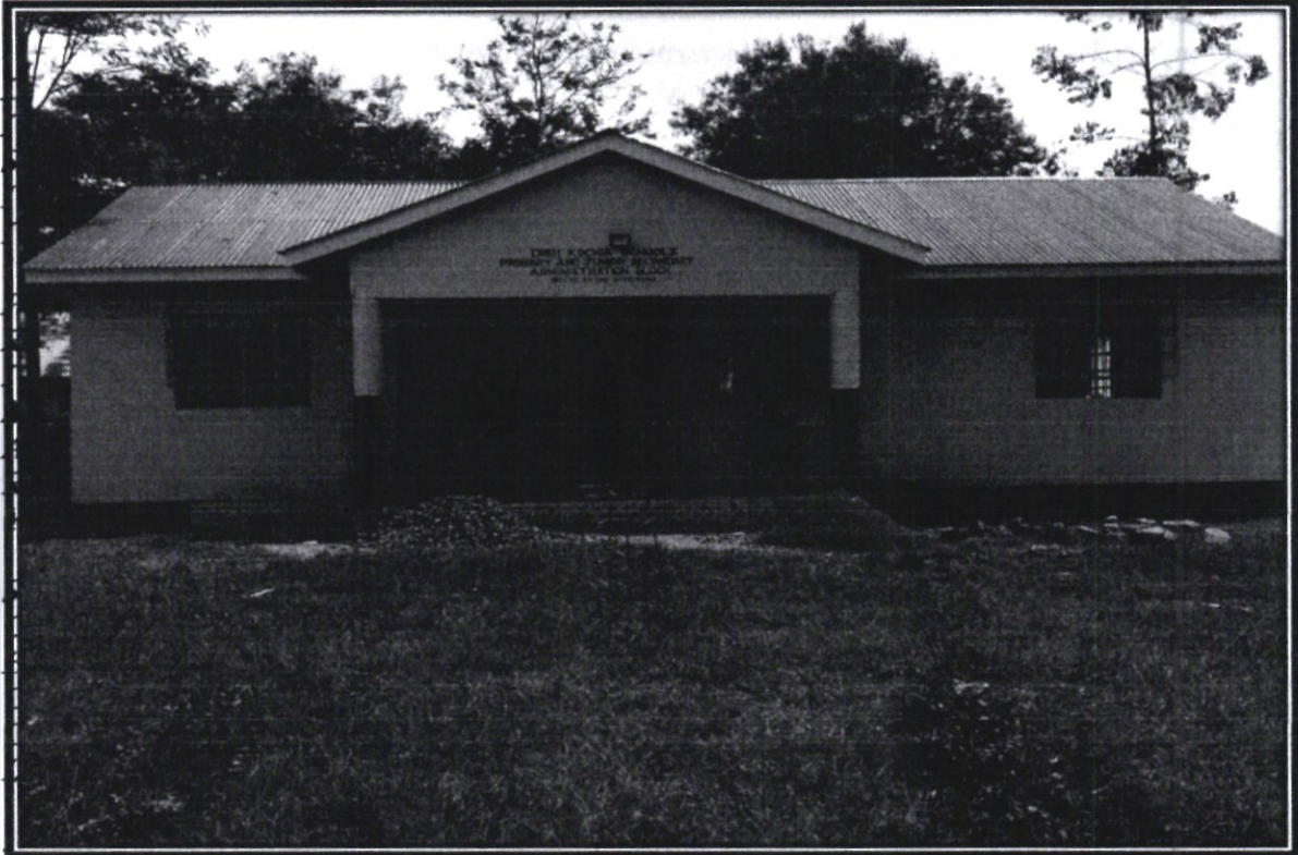
CONSTRUCTION OF AN ADMINISTRATION BLOCK.
