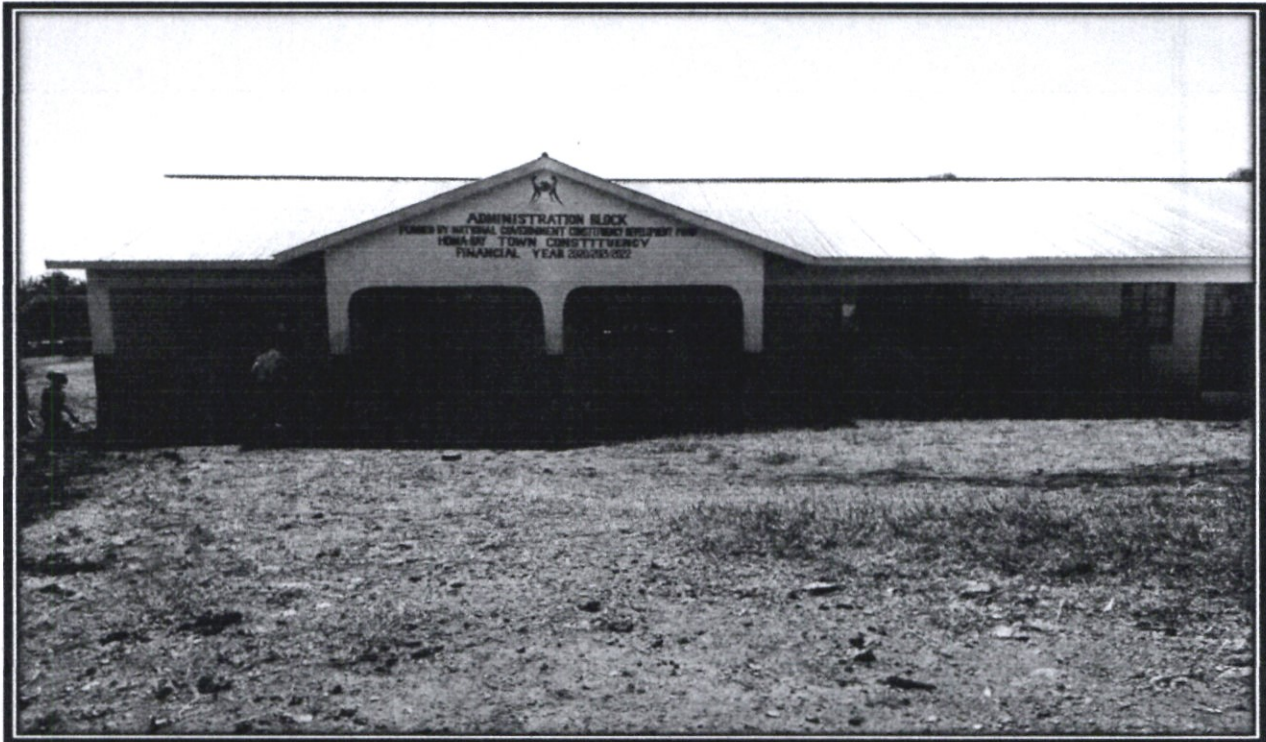
RODI PRIMARY SCHOOL: CONSTRUCTION OF AN ADMINISTRATION BLOCK.
