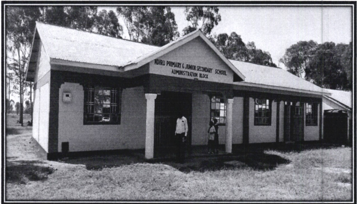
NDIRU PRIMARY SCHOOL: CONSTRUCTION OF AN ADMINISTRATION BLOCK
