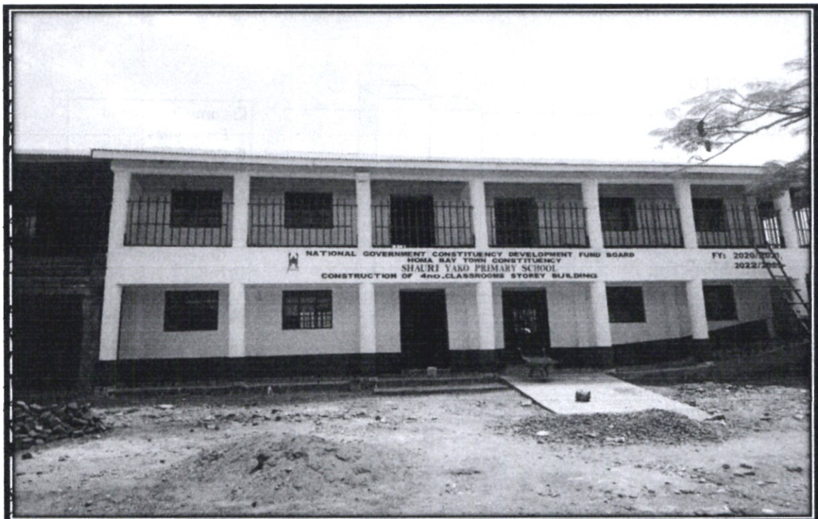
HOOL: CONSTRUCTION OF 4 NO. CLASSROOMS STOREY BUILDING
