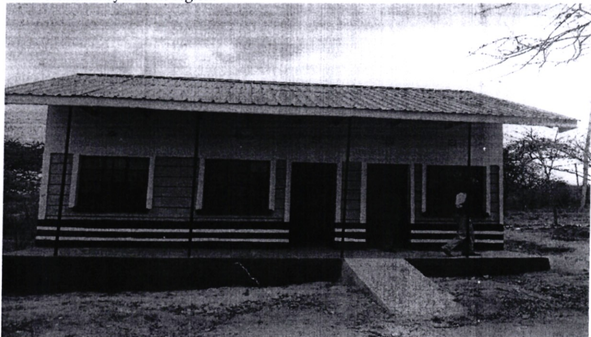
Construction of Kathuma Assistant Chief's Office going on
