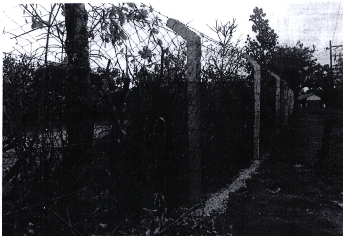
Fencing of Kyeng'e primary school
