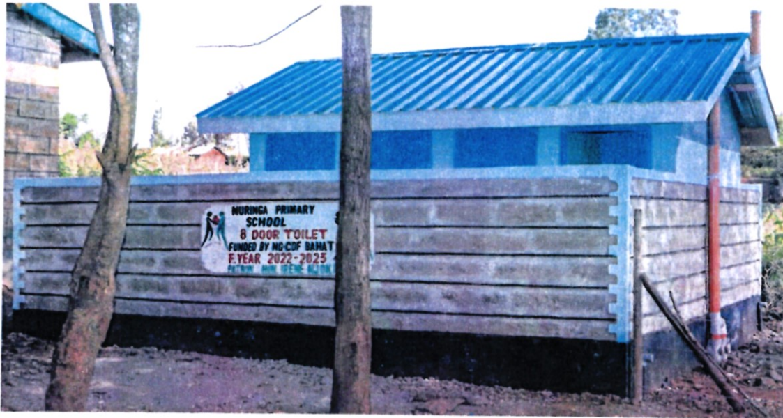
Figure 3 Muringa Primary school toilet block
