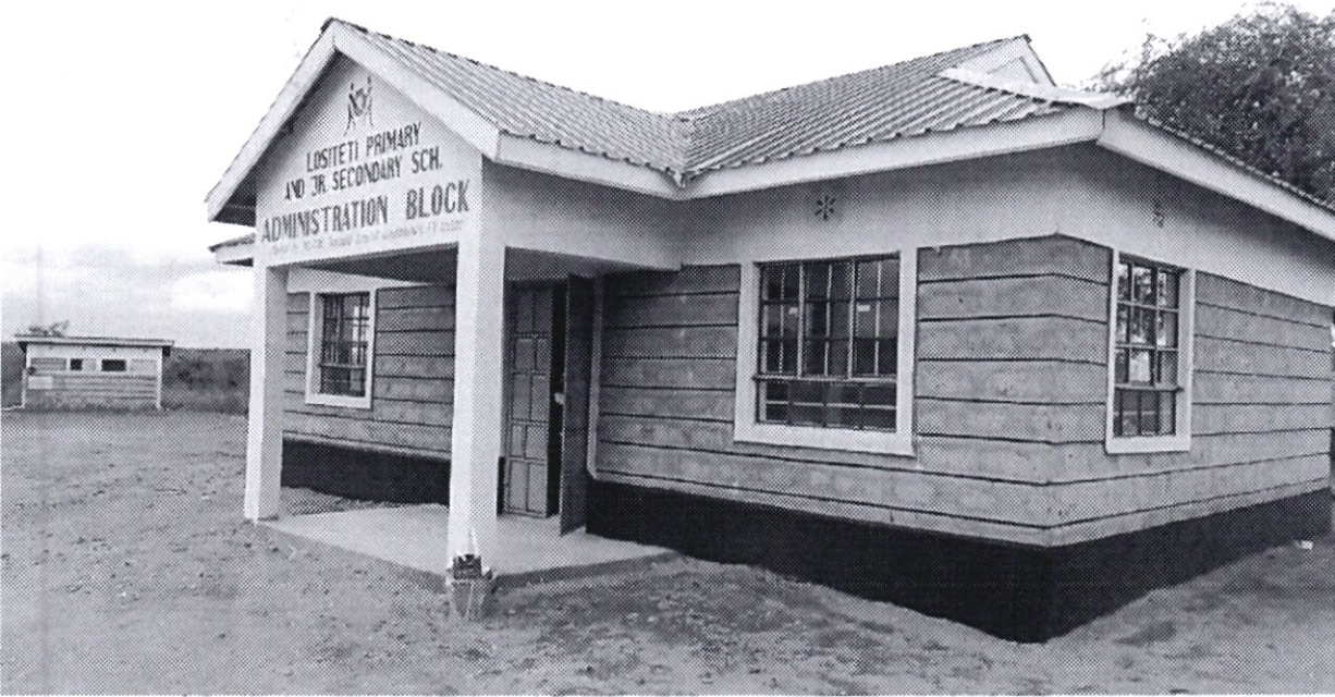
Fig 3: Lositeti Primary School Administration Block
