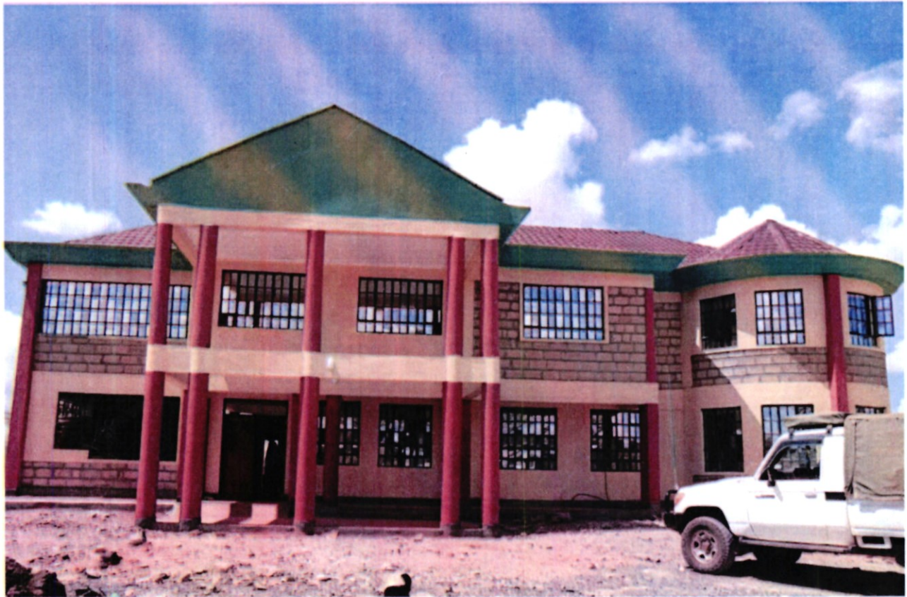
Figure 1: Ongoing Construction of NG-CDFC office at Laisamis Sub County HQ
