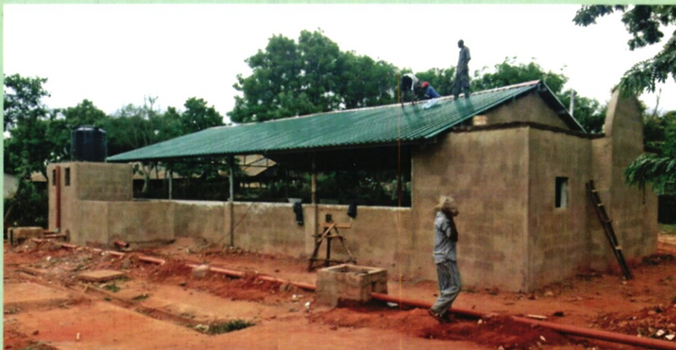
Side view of the Manyani Prison Camp Mosque under construction.
