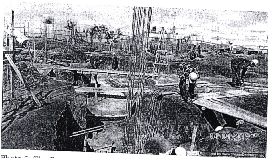
Photo 6: The Proposed County Headquarters under construction in Kathwana.
