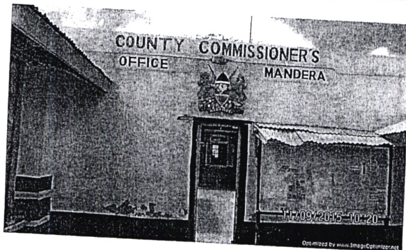
Photo 28: Manderu County Commissioner's office housed in a police station together with the security teams.
