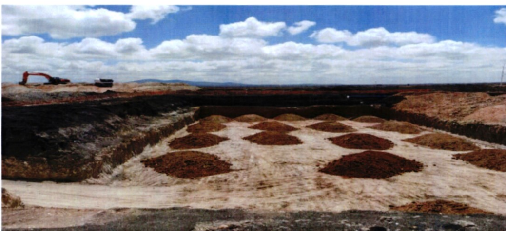
Backfilling at the Solid Waste Sorting Facility.
