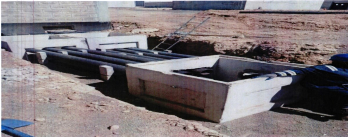
Laying of LV Network at the Water Treatment Plant
