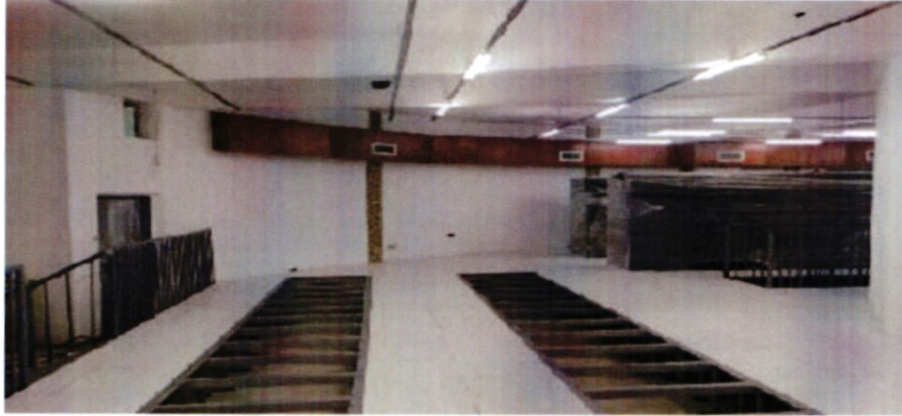
Construction of Data Centre Disaster Recovery Centre
