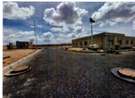
Priming of road surface at WRF roads
