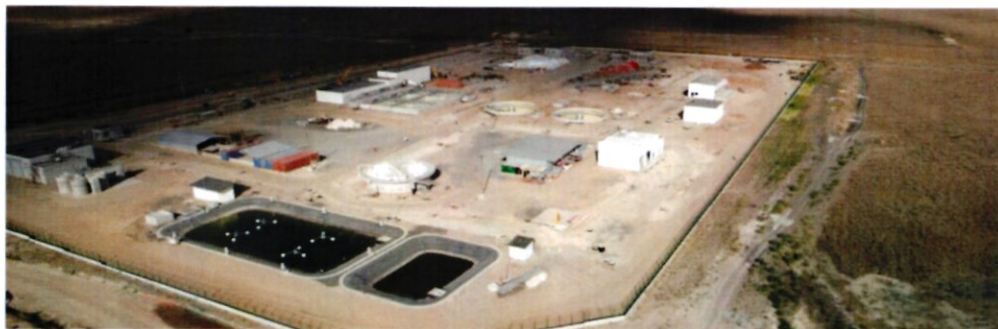
Ariel view of the Wastewater Reclamation Facility
