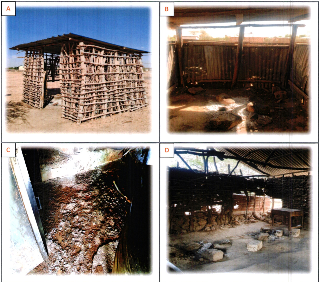
Photo A: Temporary Kitchen structure at Kone Primary School, Balambala Sub County, Garissa (31 January, 2023)
