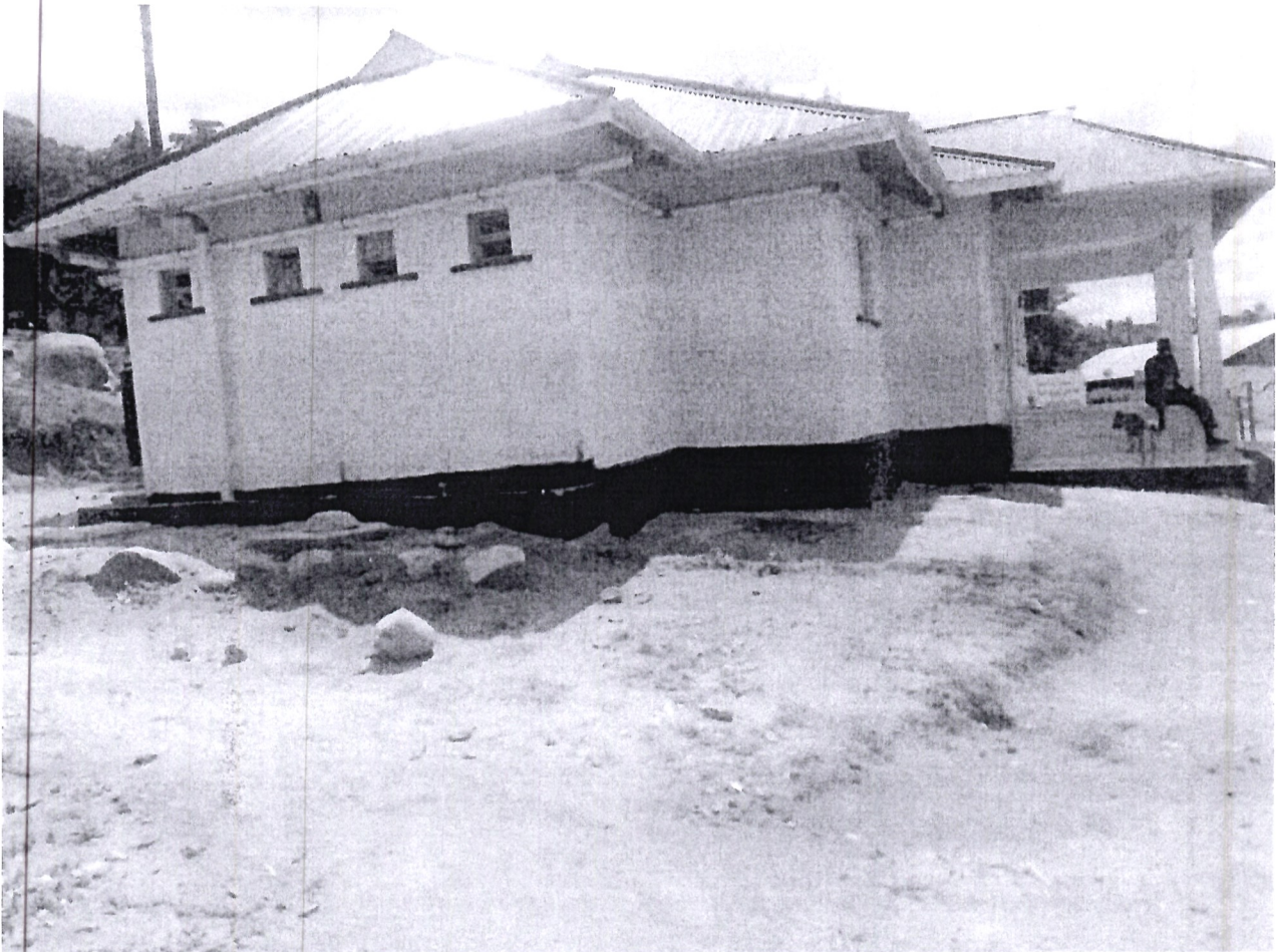
Figure 4 KOMOTOBO MIXED SECONDARY SCHOOL ADMINISTRATION BLOCK
