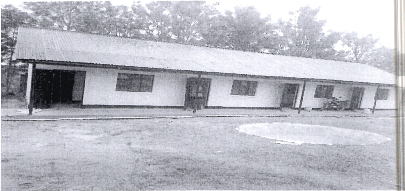
Figure 5 KOROMANGUCHA AP LINE FOUR STAFF QUARTERS
