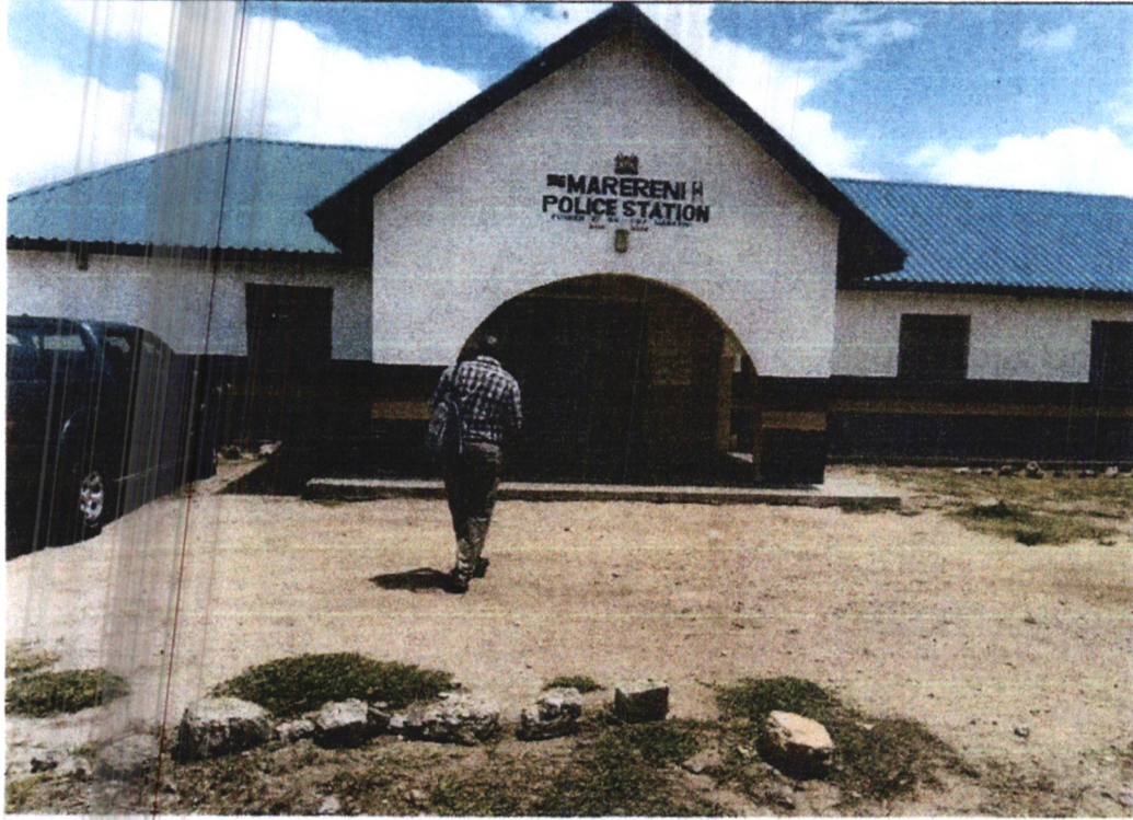
Marereni police station...Adu Ward
