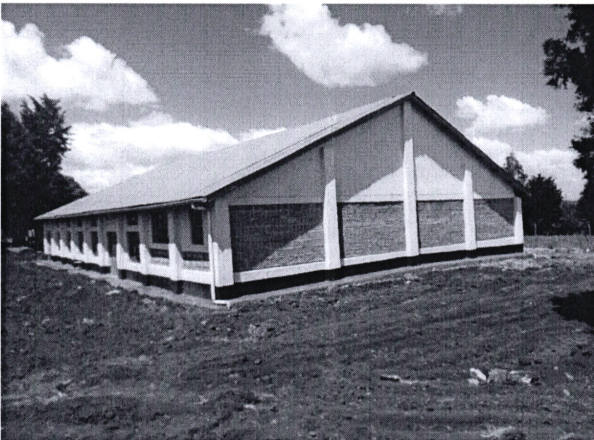
St Brigita Girls Construction of Dinning Hall Implementation challenges
